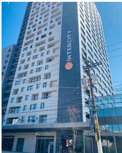
Figuras 3 – Fachada do Hotel (Intercity)
